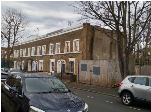
25-35 Balcorne Street. The fence for Orchard School is adj to no 25.
